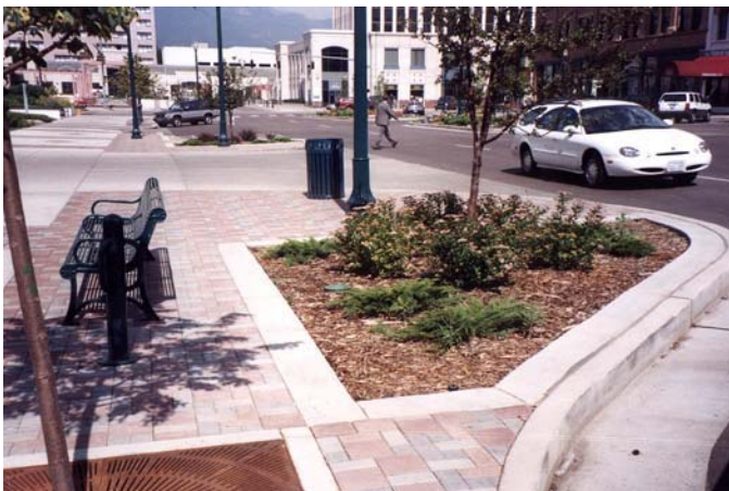
Figure 3 Colorado Springs, CO – Curb extension with driveway - the design provides a place for drivers to wait for a gap in traffic without blocking pedestrians.
