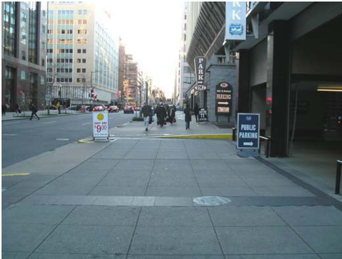
Figure 2 Washington, D.C. – Note the yellow curb across the sidewalk – a trip hazard.
