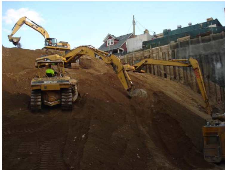
Mass excavation of soils operations.
