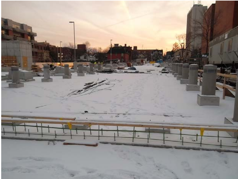
Installation of the light poles and plaza level light fixtures
