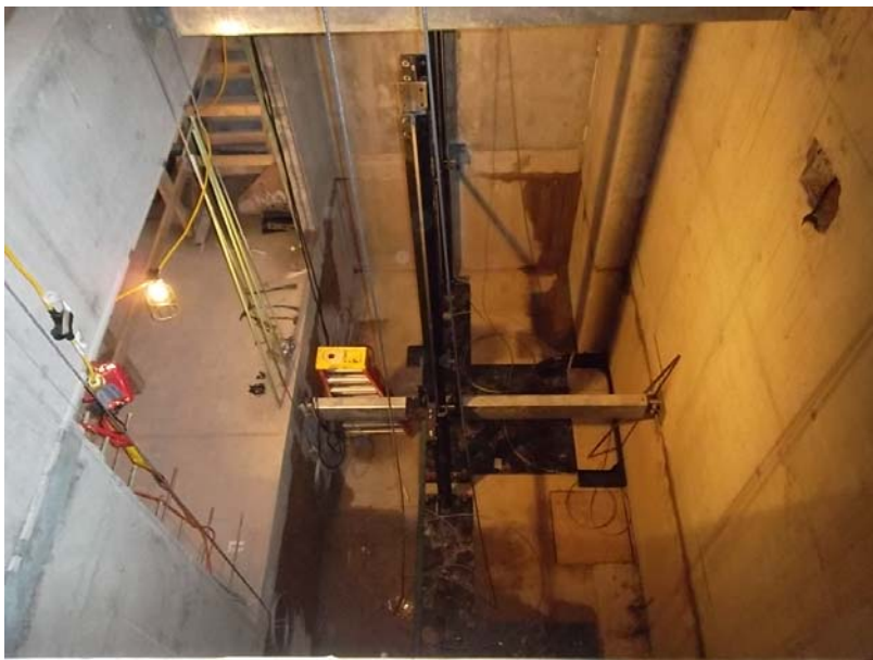
Installation of the Plaza Elevator.
